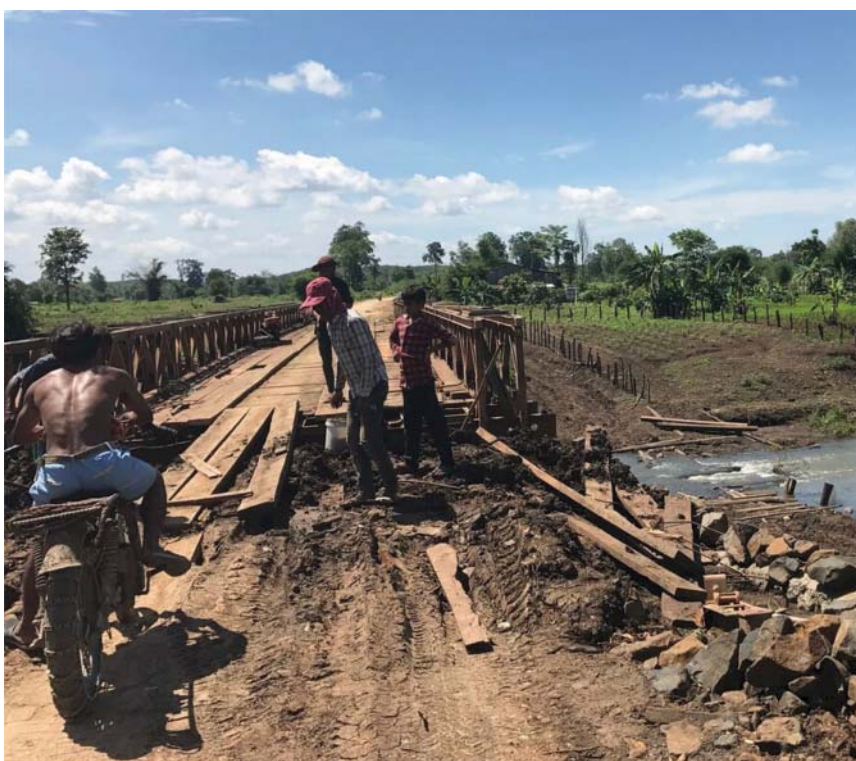
New construction driving change in Keo Seima Wildlife Sanctuary (Photo: Rebecca Riggs)
