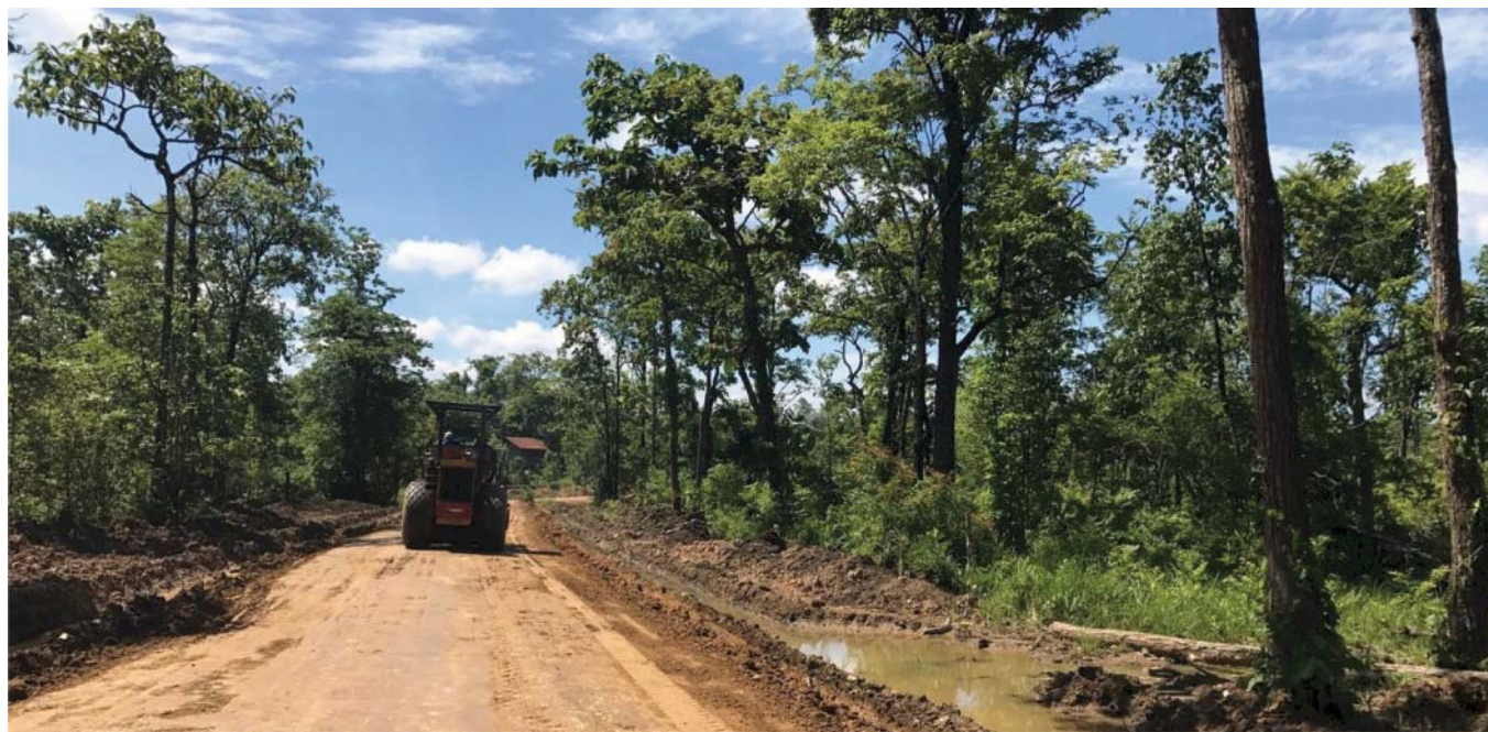
Road building inside Keo Seima Wildlife Sanctuary (Photo: Rebecca Riggs)
