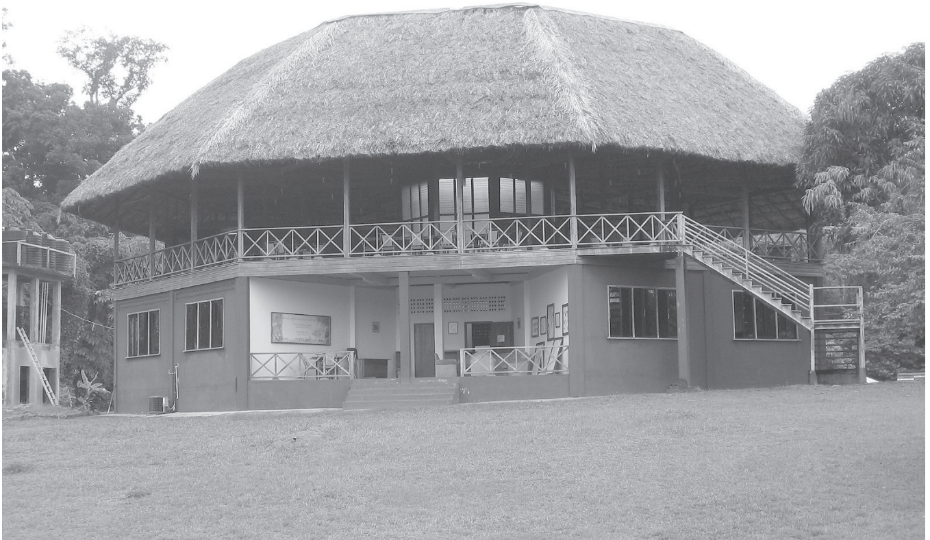
The Fred Allcock Training Centre at the Iwokrama Field Station.
